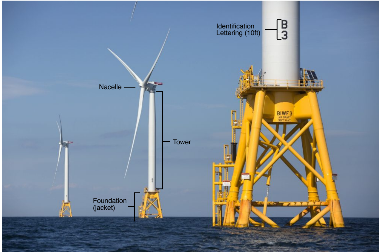
Photo courtesy of Ørsted with edits by RODA. BIWF turbines are 6MW with black lettering.
